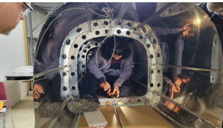
Photo showing Manu (C) inside the tail cone drilling out rivets as part of the Service Bulletin repair and Steve (L) providing assistance and moral support. Photo credit: R. Montero
